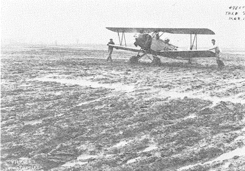
A good argument for hard surfaced runways. With few exceptions, elementary flying was done from grass covered fields which were safer and easier for beginners. When this field at No. 9 EFTS at St. Catharines become too muddy in March 1941 flying was temporarily transferred to No. 16 SFTS at Hagersville. (PMR 75-353) F. Pattison photo.
